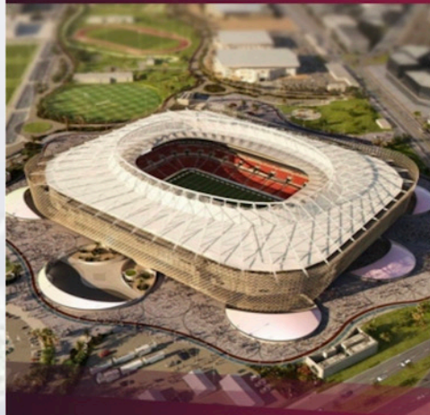
AL RAYYAN STADIUM AL RAYYAN
